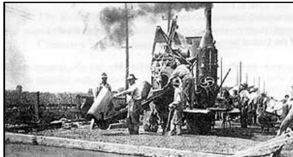
The concrete was mixed and poured on the job site.
